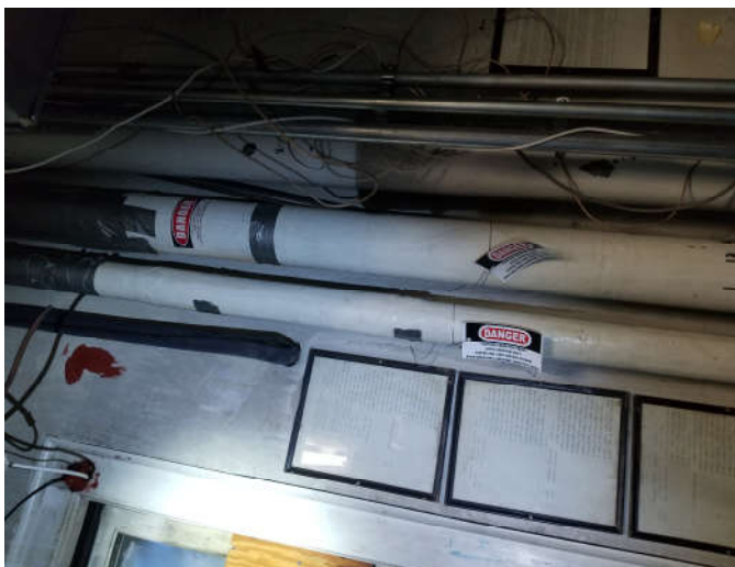
b1 room a4 pipe insulation
