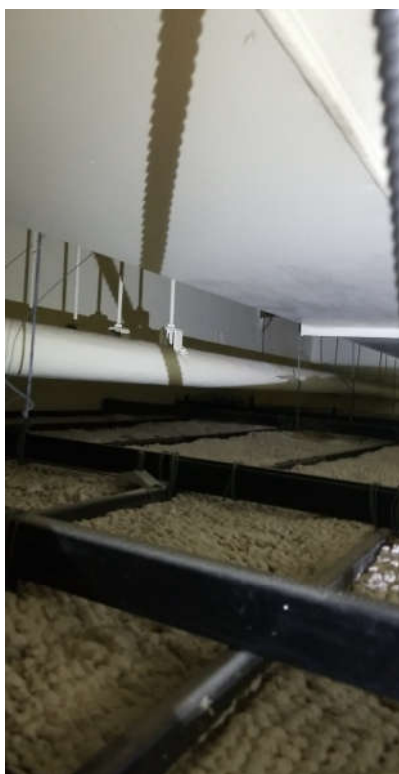
ph stairwell pipe insulaion
