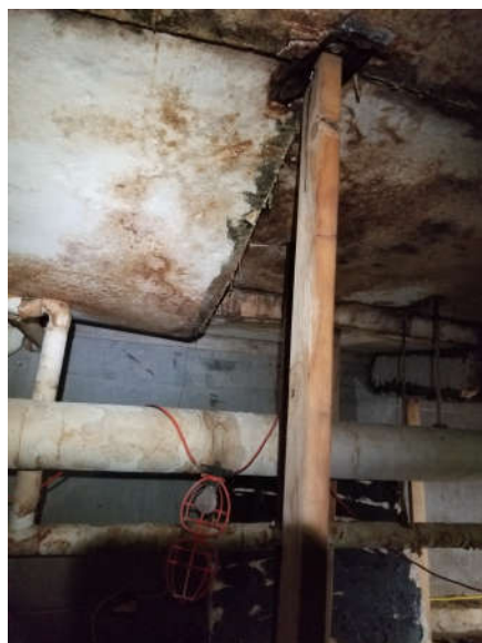
crawl space styrofoam with black mastic 3
