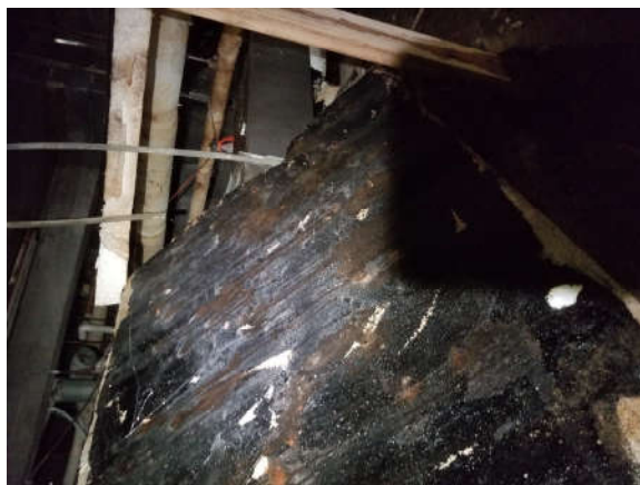
crawl space styrofoam with black mastic 2
