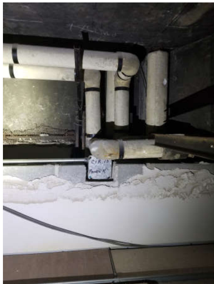
basement room a25 pipe insulation
