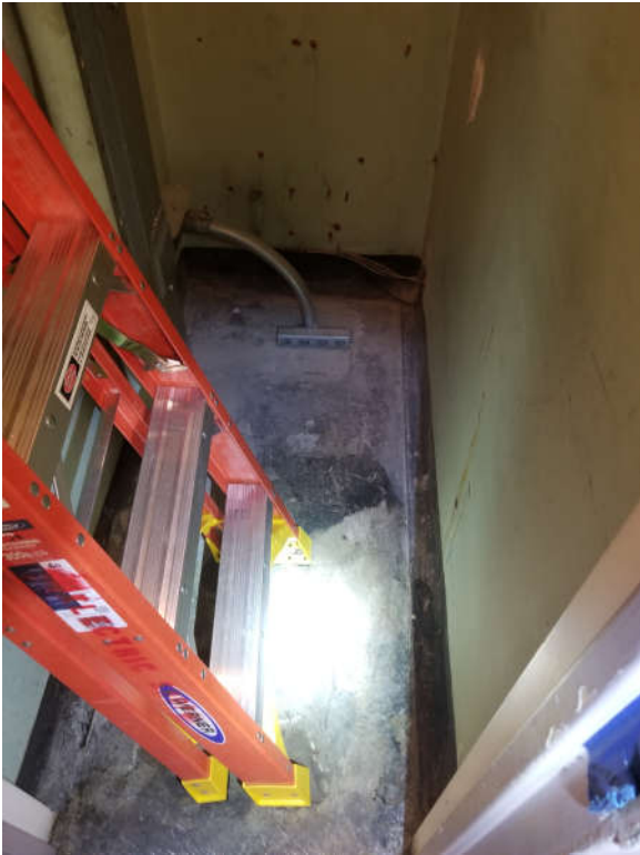
9th Floor hallway
