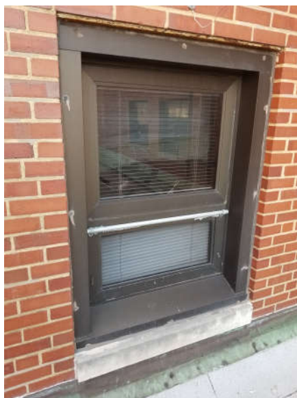
exterior window caulking
