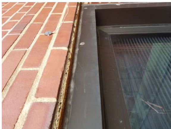
exterior window caulking 2
