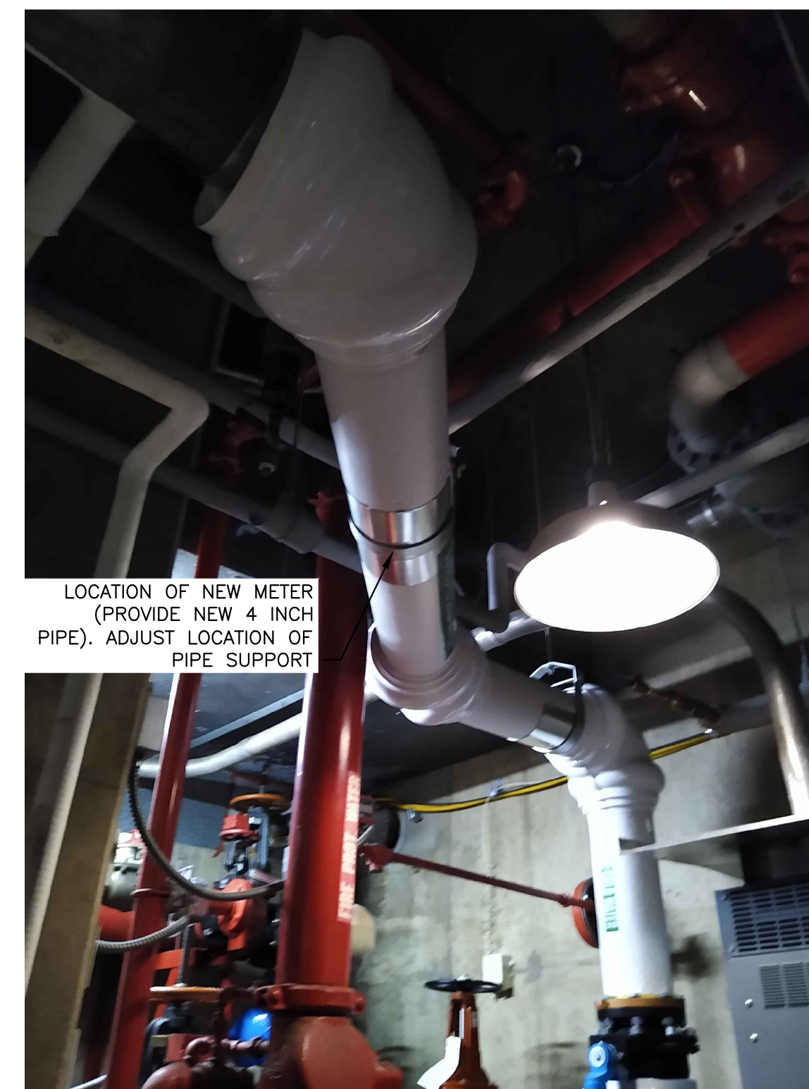
4 DM WATER GENERAL LOCATION P-13 Scale: NONE (PHOTO)
