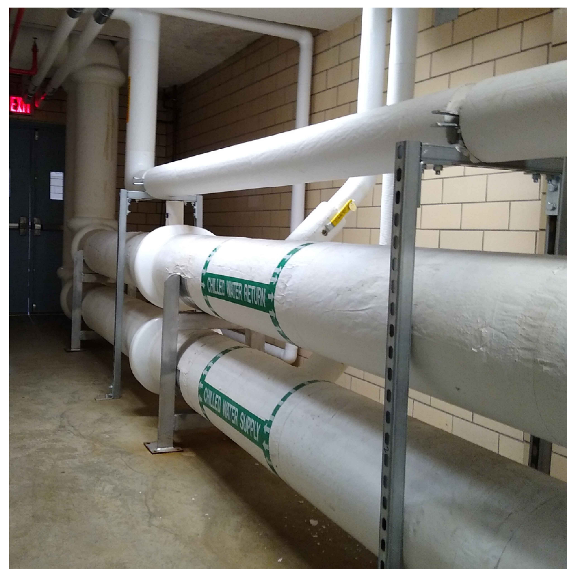
5 M-2 PHOTO: CHILLED WATER EXISTING CONDITIONS No Scale
