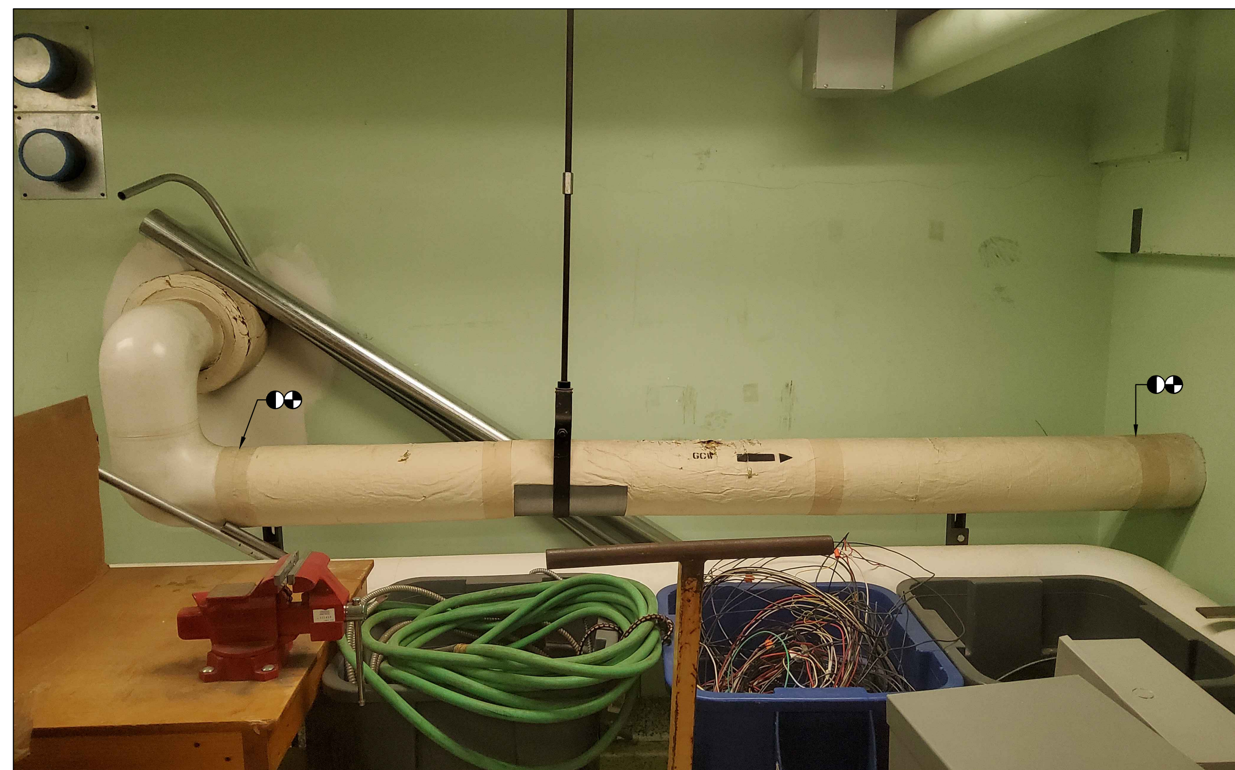
2 PHOTO: DOMESTIC WATER METER LOCATION P-8
