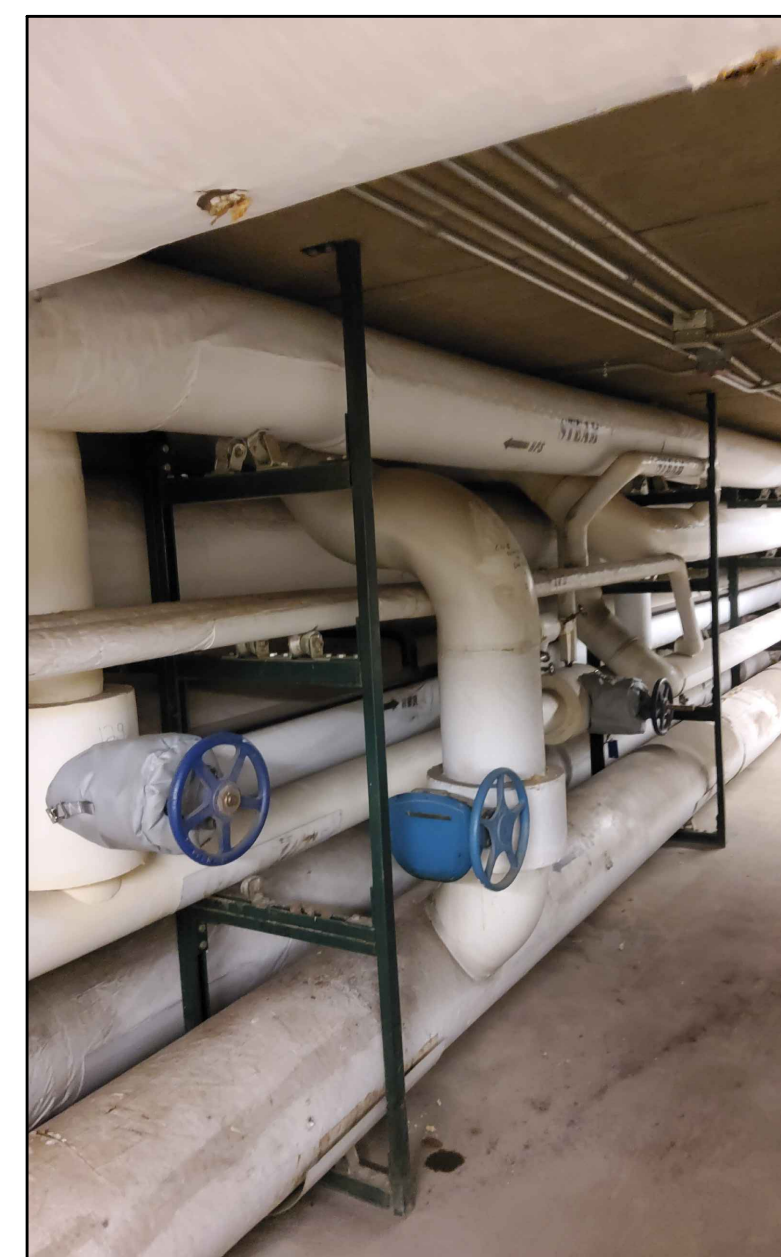
7 PHOTO: SOUTH CHWS Scale: NONE SERVES EAST BLDG
