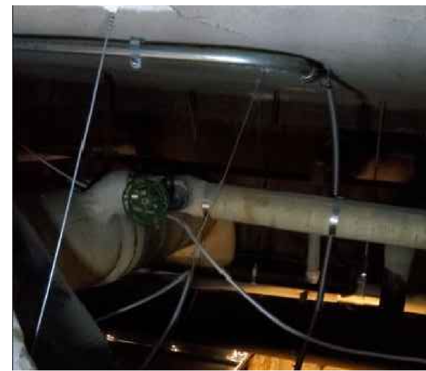
2 PHOTO: STEAM PIPE WORK (AOW) Scale: NONE NORTH 2 INCH MAIN
