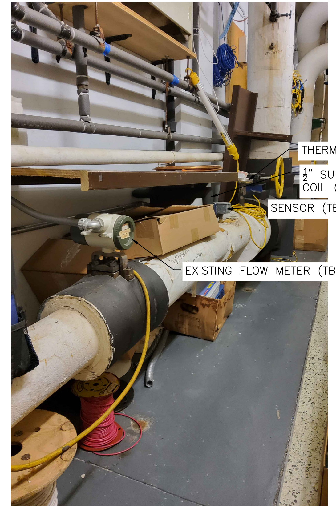
3 PHOTO: LOCATION OF NEW CHWS METER M-8A NOT TO SCALE NOB-CHWS-M01
