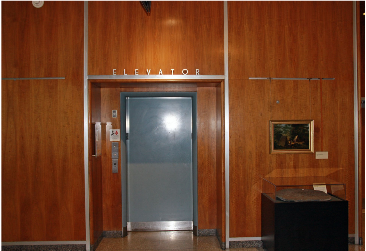
Photograph 5 Walnut veneer paneling and terrazzo floors at the Ground Floor.
