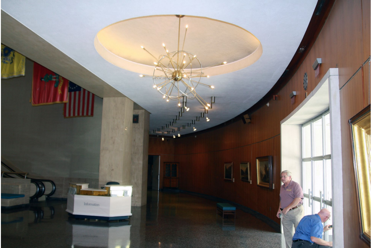
Photograph 1 Ornamental chandelier, terrazzo floor, travertine wall and walnut veneer wall panels at Lobby M115.
