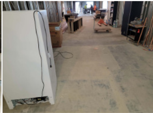
Building 4 Overview 1 st Floor (Near 1B53)
