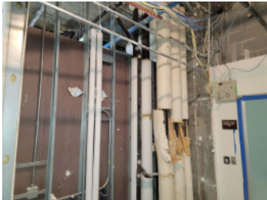
Building 4 Overview 1 st Floor (Near 1B53)
