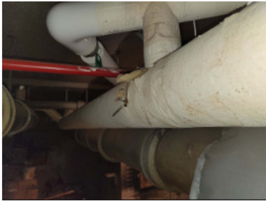
Basement TSI Overview
