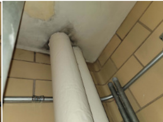
Room 1D22 Overview
