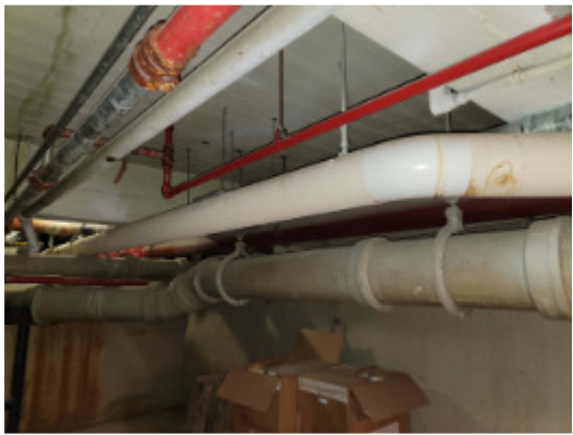
Basement TSI Overview
