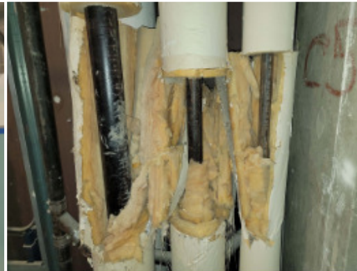
Building 4 Overview 1 st Floor (Near 1B53)
