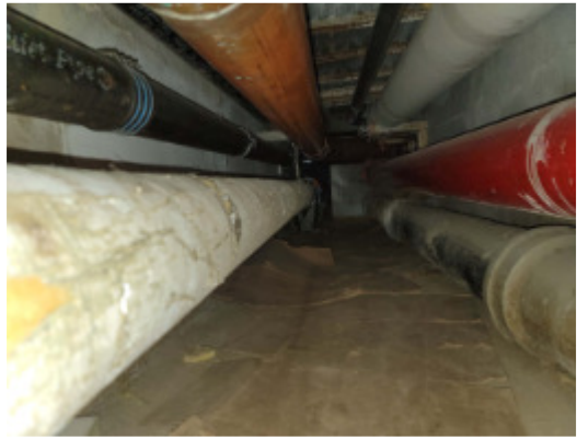
Basement TSI Overview
