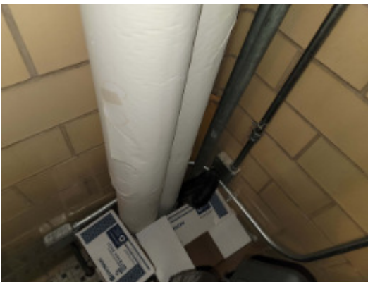
Room 1D22 Overview
