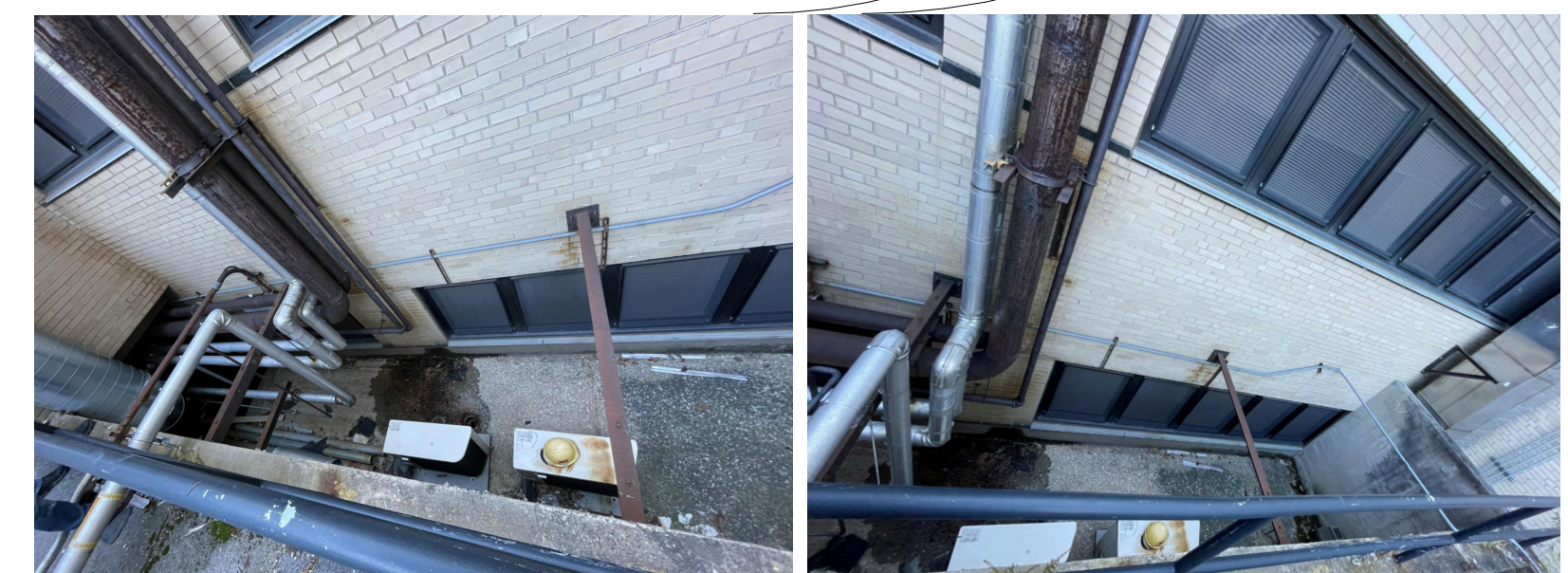
PHOTOS OF POSSIBLE CONTRACTOR ENTRANCE FOR LARGE PIPE SECTIONS SHOWN FOR REFERENCE ONLY.
