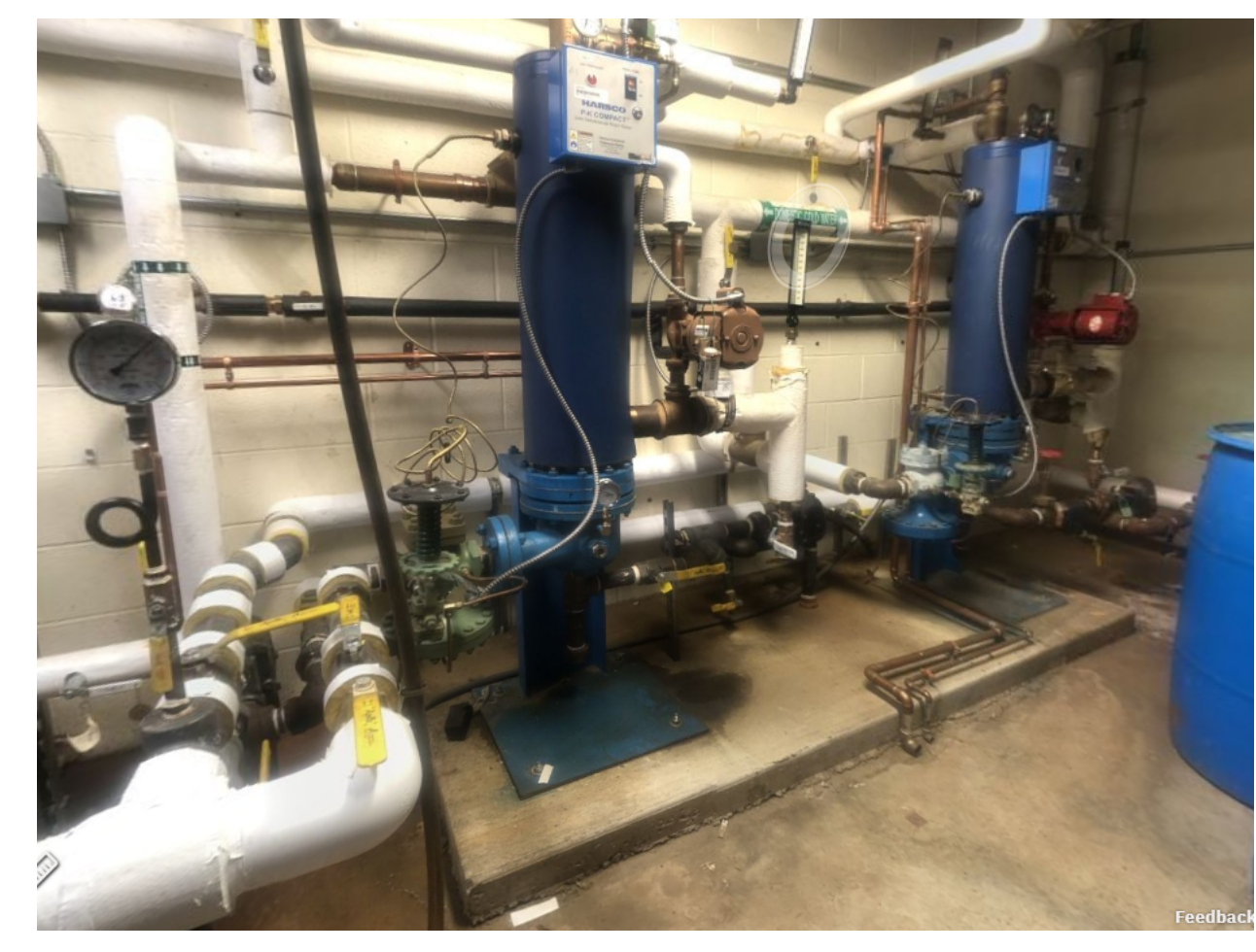
2 BD01B - DOMESTIC WATER HEATER NTS
