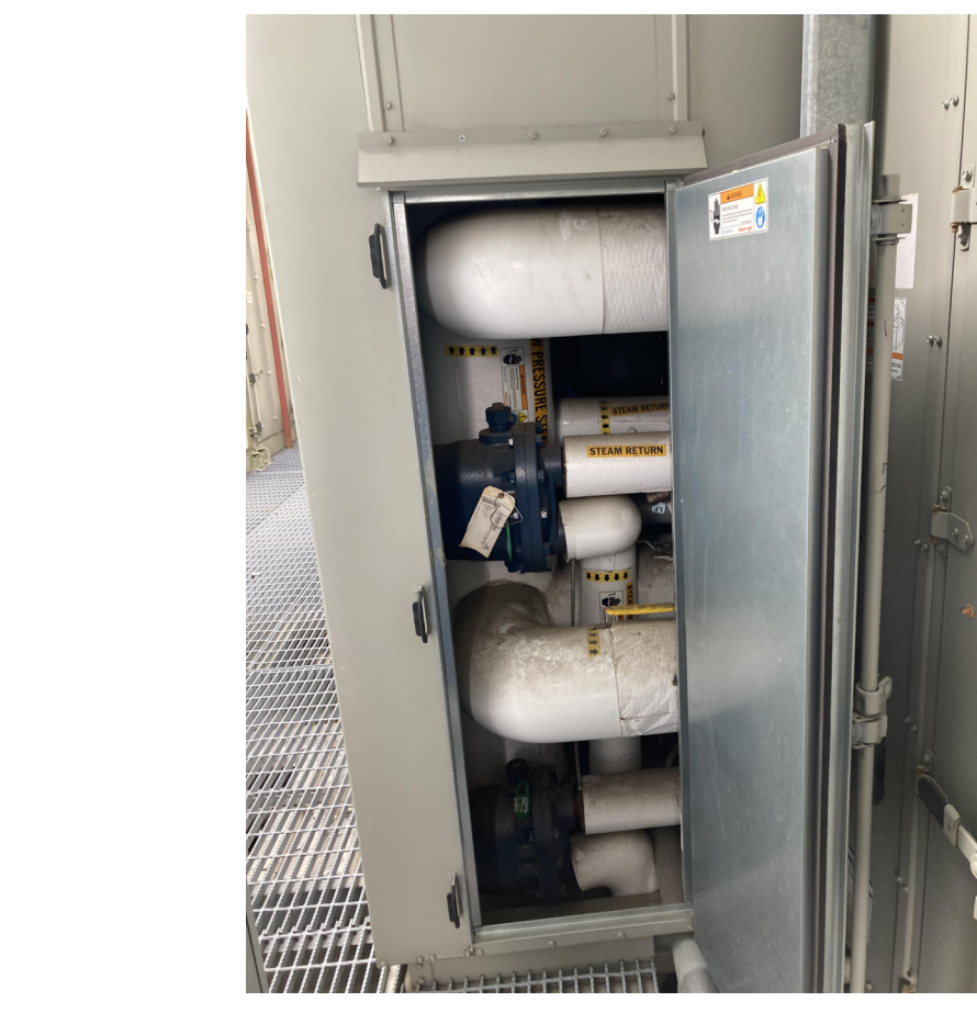
2 RTU - 1A - TRAPS NTS
