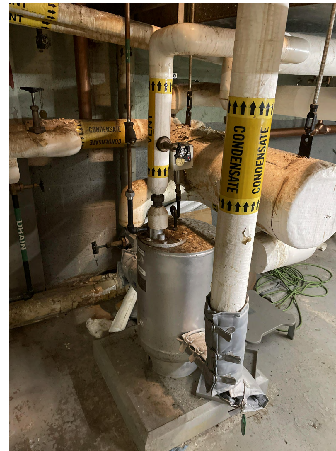
5 MECHANICAL ROOM BB12 - EXISTING CONDENSATE PUMP NTS
