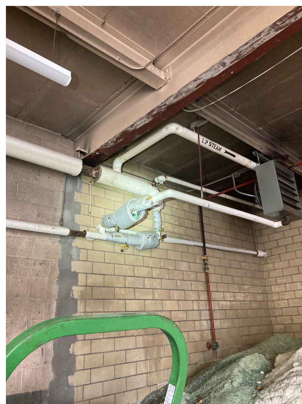
1 BUILDING 3 UNIT HEATER TRAP #1722 NTS
