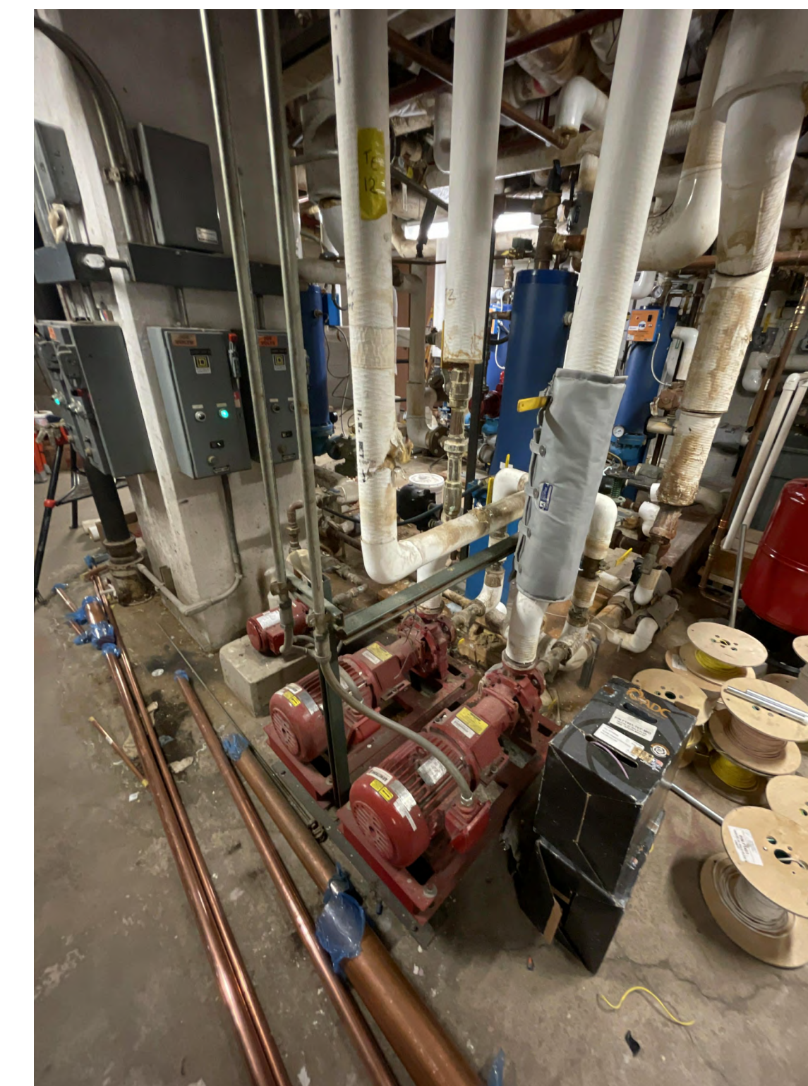
2 MECHANICAL ROOM BA10 - EXISTING DOMESTIC PUMPS AND HEATERS NTS
