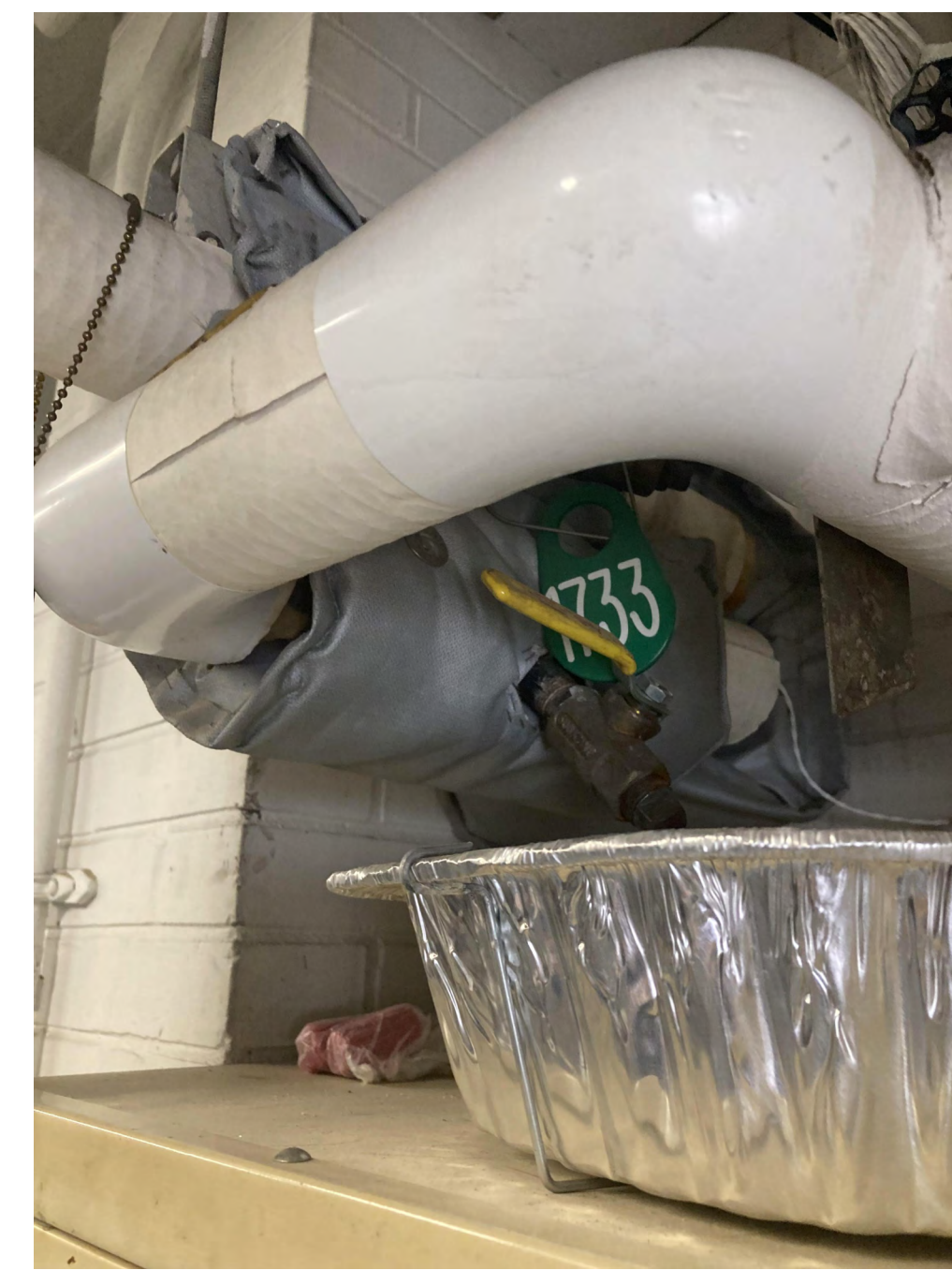
2 BUILDING 3 END OF LINE TRAP #1733 NTS
