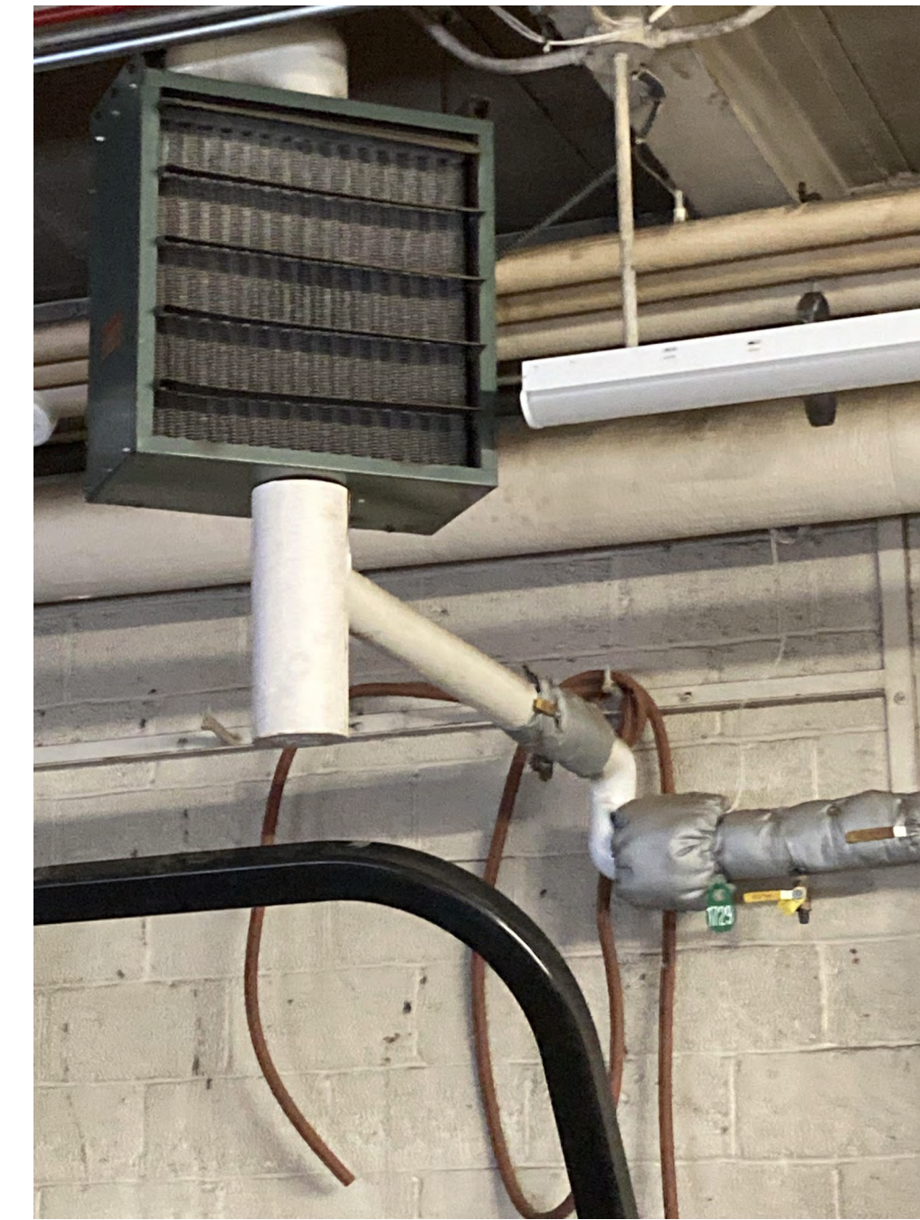
3 BUILDING 3 UNIT HEATER TRAP #1729 NTS
