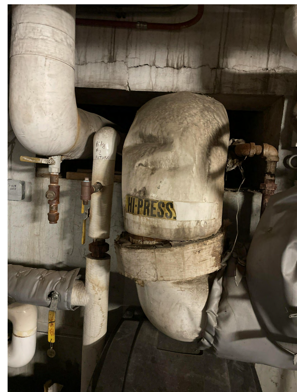
6 MECHANICAL ROOM BA10 - EXISTING CONDENSATE LINES NTS
