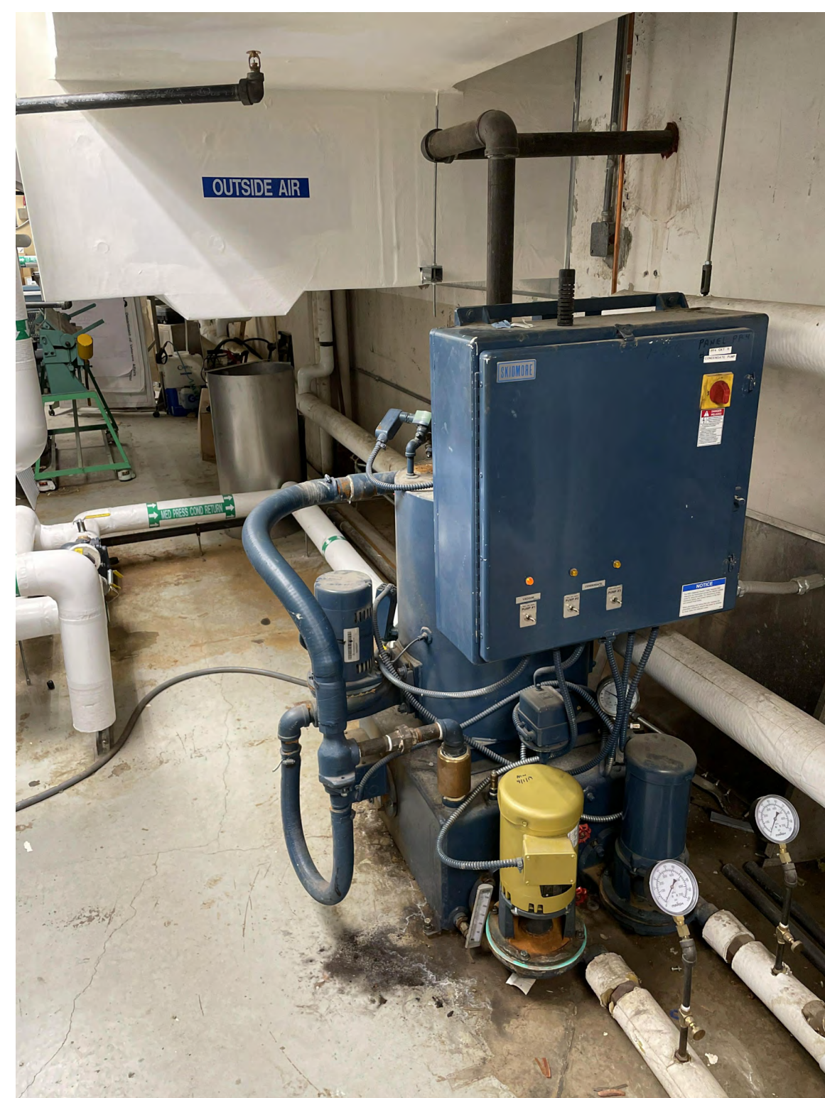
9 MECHANICAL ROOM BC11 - EXISTING CONDENSATE PUMP NTS
