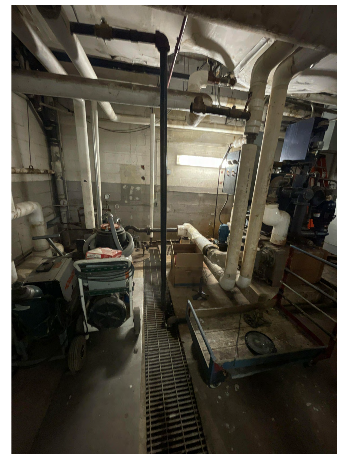
4 MECHANICAL ROOM BA10 - EXISTING STEAM PUMPS NTS
