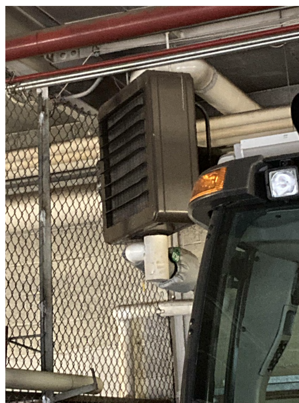
4 BUILDING 3 UNIT HEATER TRAP #1730 NTS
