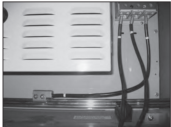
4. Remove the orange insulation and install the bussbar for line 3 (back). Connect lug for line three on each module.
