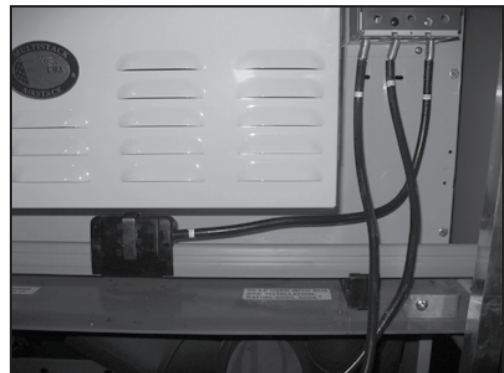
6. After connecting the lugs for line three of all the modules, cut the orange insulation to fit between the lugs. Now install the lug cover and snap the bussbar into place on the plastic holders.
