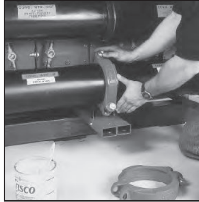
8. Starting with the lower header, install the couplings. Position coupling bolts as shown in order for proper installation of frame. (Bolts @ 1:00 and 7:00)
