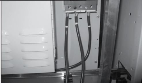
3. Install the three bussbar connector wires to the isolation switch to each Heat Pump. The wires are shipped with each module and are tied to the compressor feet on each module.
