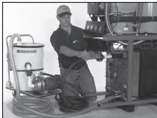
Figure 3, Inserting FlushGun into heat exchanger.
