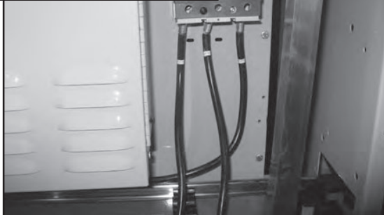
3. Install the three bussbar connector wires to the isolation switch to each Heat Pump. The wires are shipped with each module.
