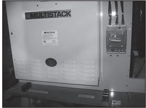
2. Remove the isolation switch cover
