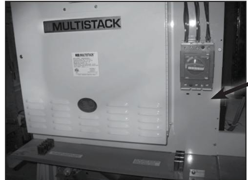
2. Remove the isolation switch cover
