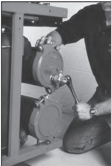
11. Install the header blank ends, start with the bottom blank B, then move to the top blank A which includes the drain valves (evaporator shown).
