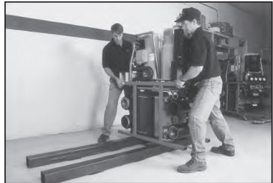
2. Slide module into position.
