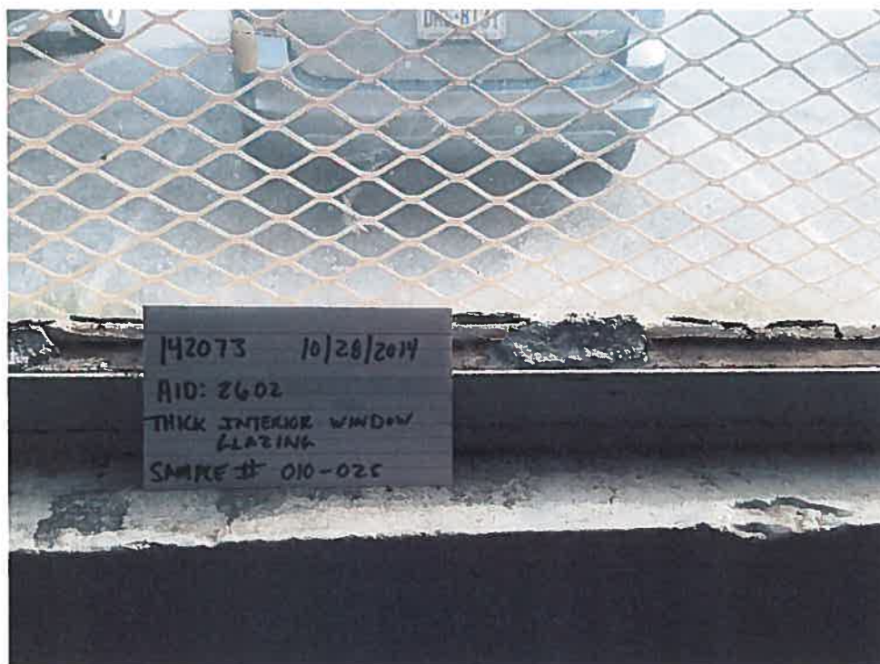
Figure 11: HID#2602 – Thick Interior Window Glazing
