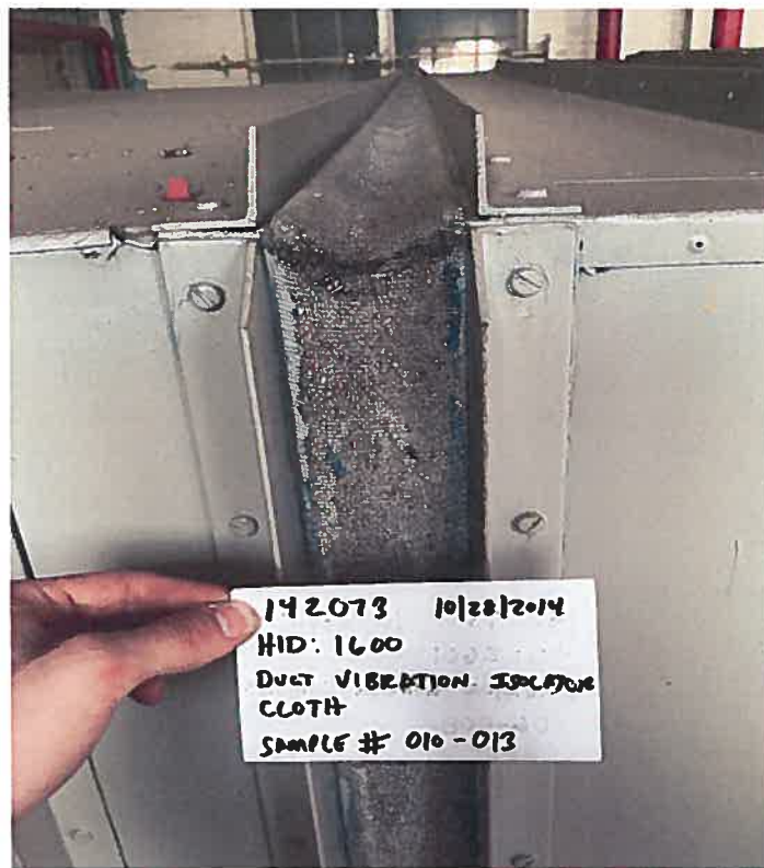
Figure 5: HID#1600 – Duct Vibration Isolator Cloth
