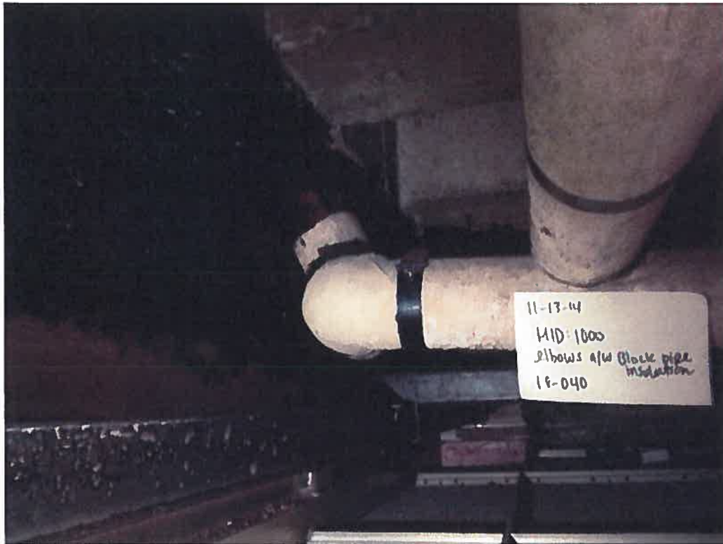
Figure 21: HID#1000 – Elbows Associated with Block Pipe Insulation
