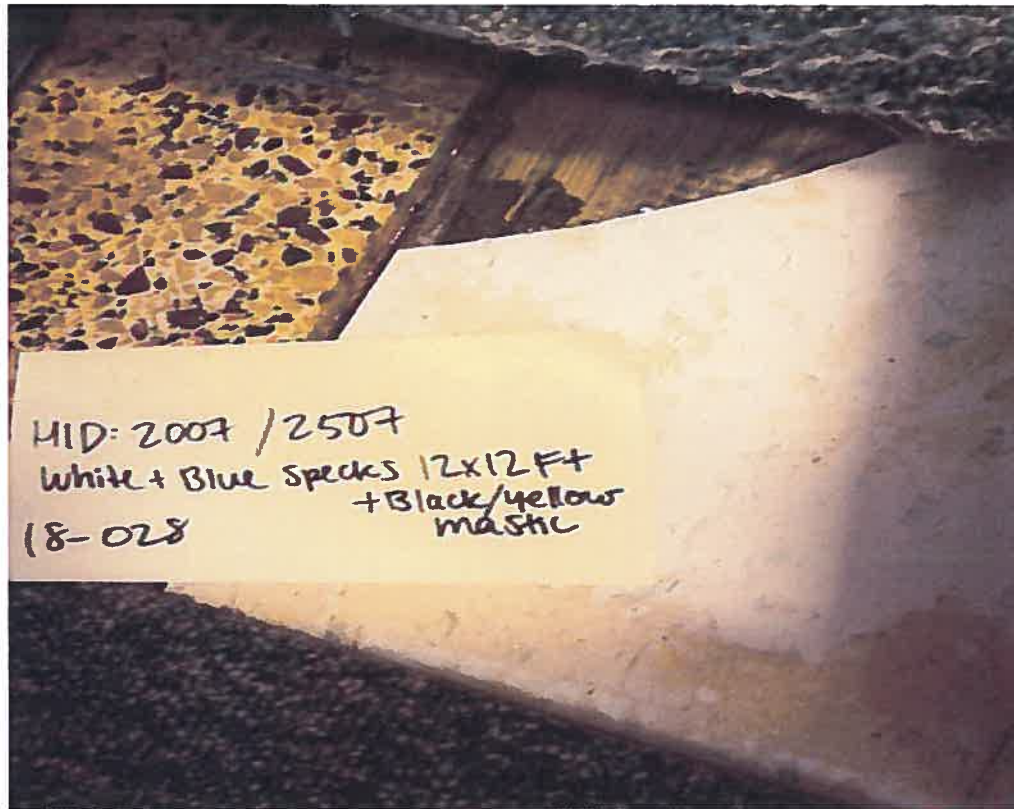
Figure 15: HID#2007/2507 – White & Blue Specks 12"x12" Floor Tile with Yellow & Black Mastic
