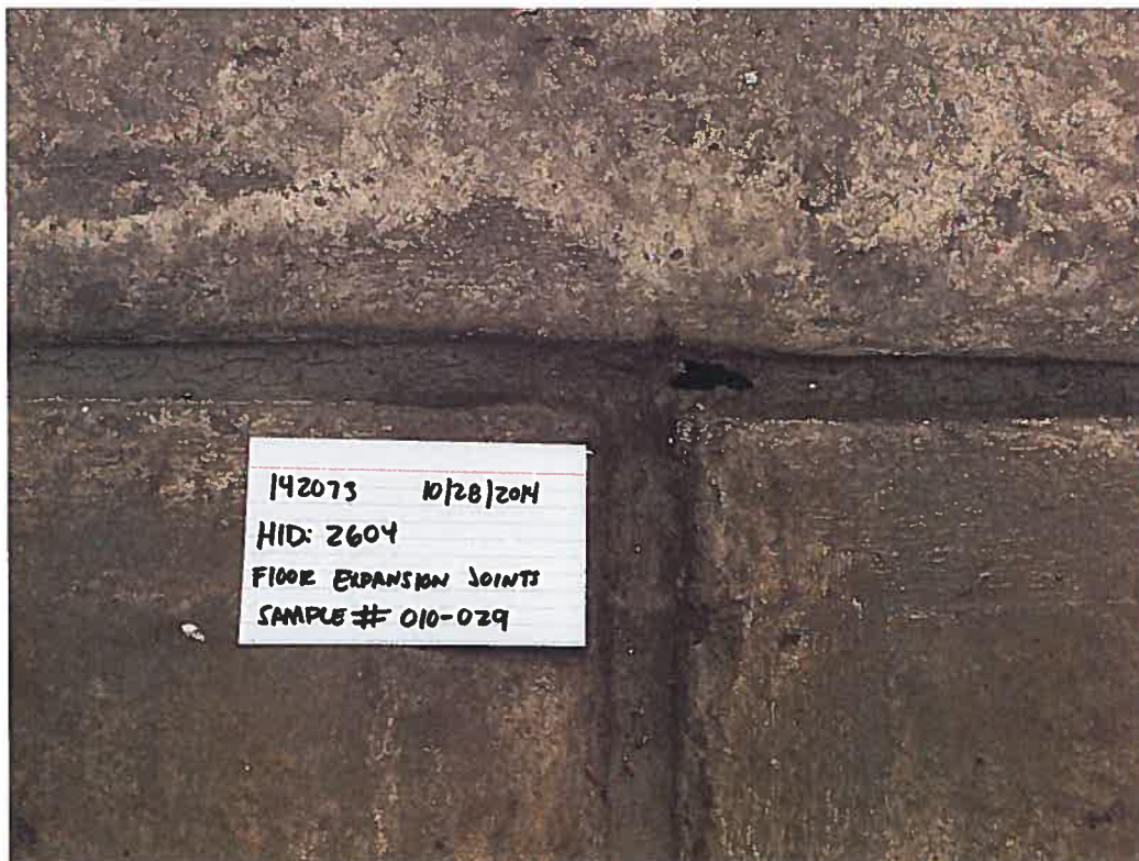
Figure 14: HID#2604 – Floor Expansion Joint
