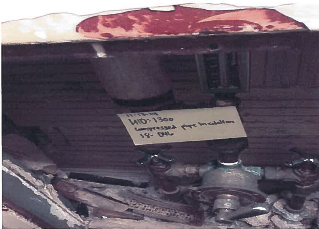
Figure 1: HID#1300 – Corrugated Paper Pipe Insulation
