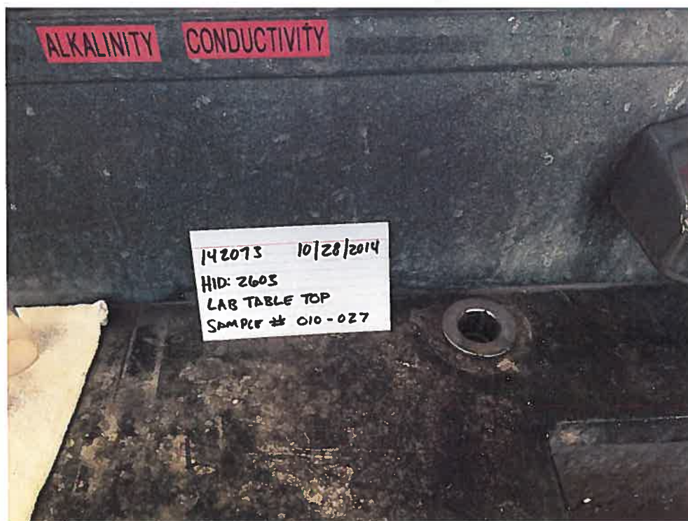
Figure 12: HID#2603 – Transite Counter Top
